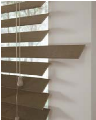
Rout hole/ center cord slat
